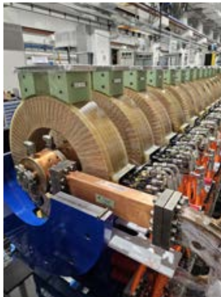
Figure 17.7: SPARC_LAB solenoid during installation at SPARC_LAB, without the iron shield upper half
